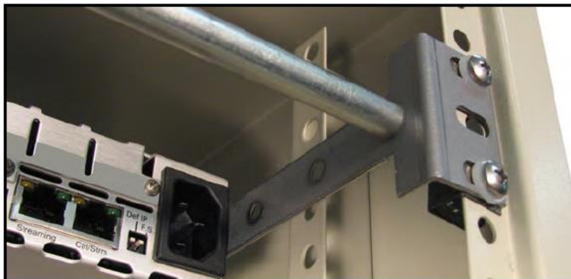
Figure 7: Installed Support Arms and Cable Relief Bar
